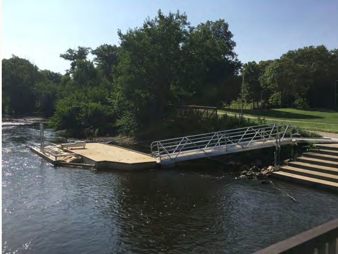
City of Lansing Project TR043 Universally Accessible Canoe/Kayak Launch at Moores Park
